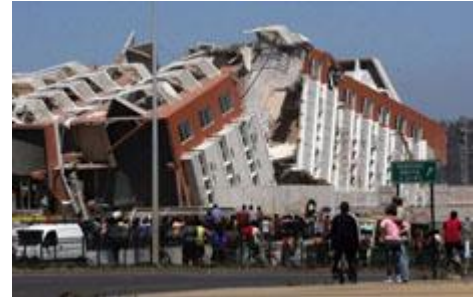
The Alto Río Apartment Failure
